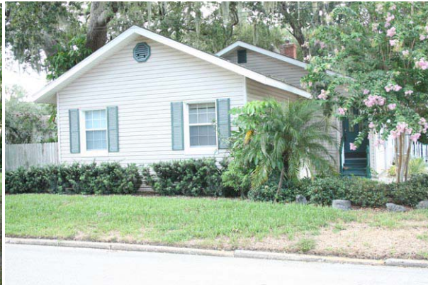
Figure 1.2 Large Gable at end with partially exposed gable where house is wider
