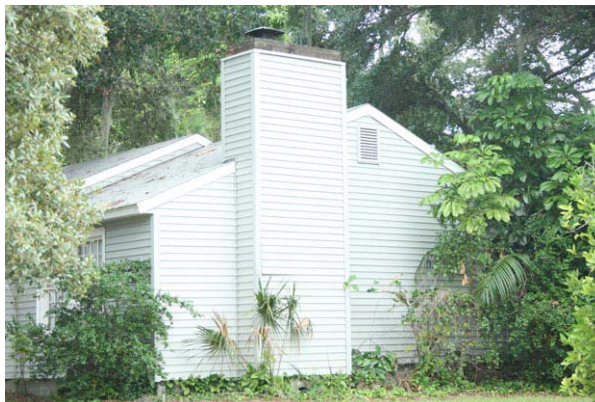
Figure 1.3 Gable end with attached chimney
