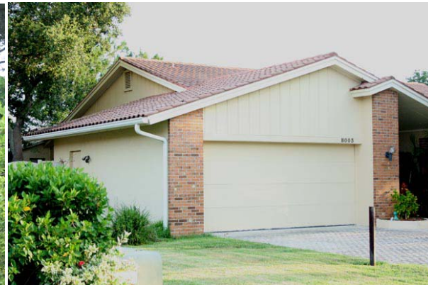
Figure 1.4 Cut off gable over garage with covered entry to side
