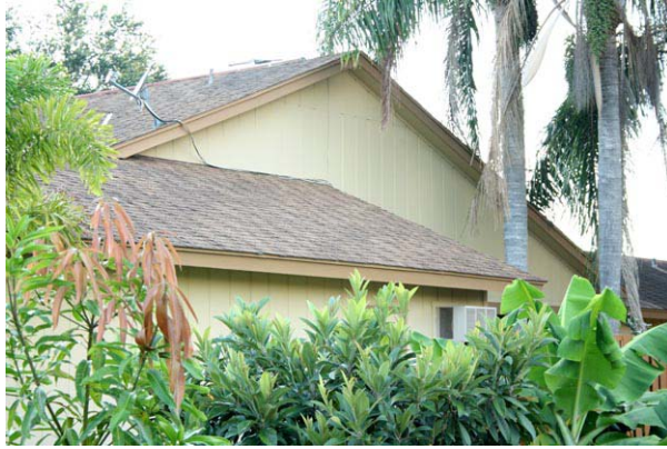
Figure 1.5 Gable end with intersecting shed roof
