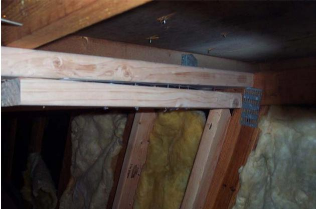
**Wrong:** Some of the fasteners for connecting the compression block to the horizontal brace do not penetrate the brace by the gap between the two.
