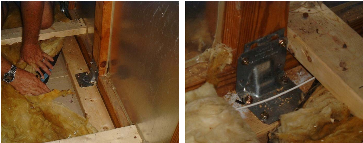
Figure 9.2. This shows an HGA installed on top of deadwood for the ceiling drywall below. It can be seen that if the HGA had not been installed on the stud of the truss, the top two screws would have missed penetrating the bottom chord. Sometimes one can drive the quarter inch screw through plates because they just happen to hit a hole in the plate. Otherwise, one needs to drill a starter hole. Doing this does not compromise the truss or the plate. From the other figures, you can see that the two outer vertical screws really are not doing much because they only penetrate the deadwood. 1-1/2" screws were used here so they did not penetrate the deadwood and the ceiling drywall. 4-1/2" screws were used for the other two so that they would penetrate the deadwood and the two top plates to make a much better connection.
