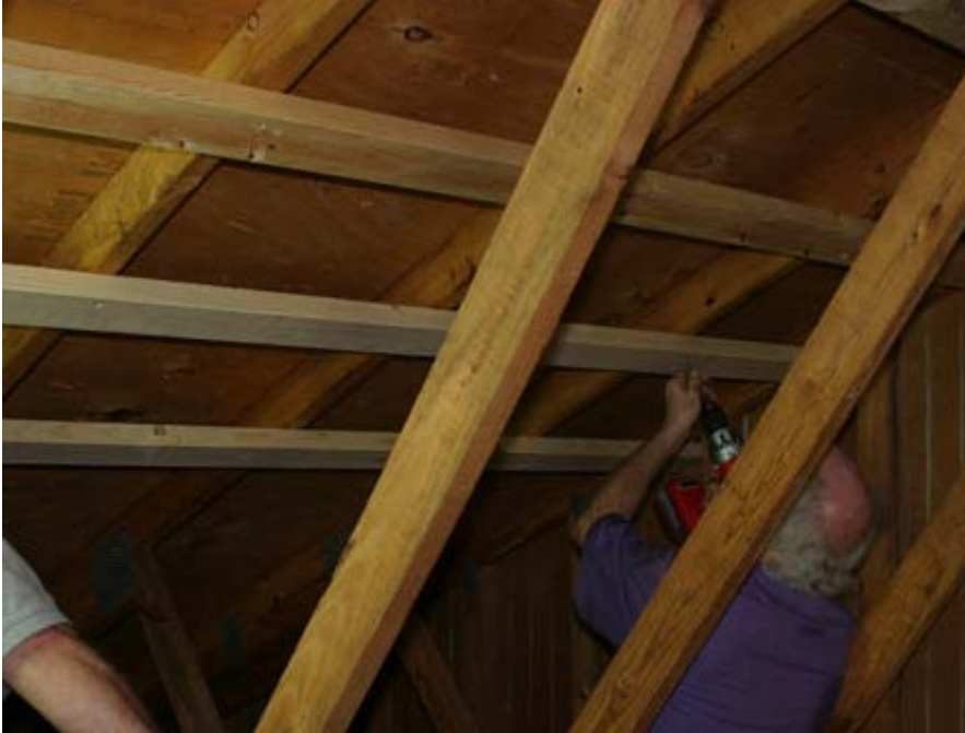
Figure 8.1. Installation of upper horizontal brace by having started screws before lifting the brace up to fasten it.
