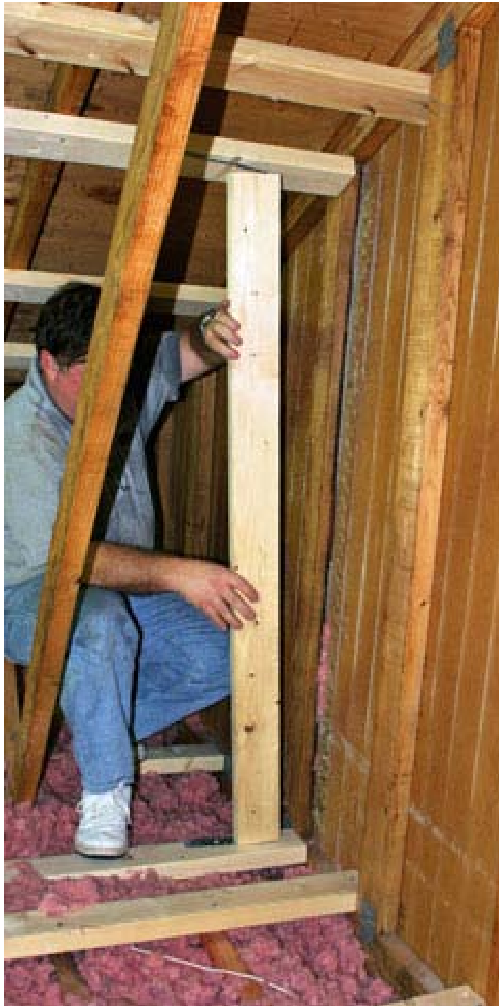
Figure 6.2. Installation of retrofit stud. The retrofit stud for this L-bent strap installation has straps already attached to the back edge. Construction adhesive has been applied to the wall where the retrofit stud will be butted.
