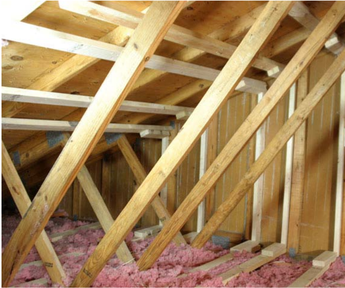
Figure 2.2 Photograph of completed gable end retrofit using the L-bent strap method – the light colored wood is the lumber added during the retrofit activity
