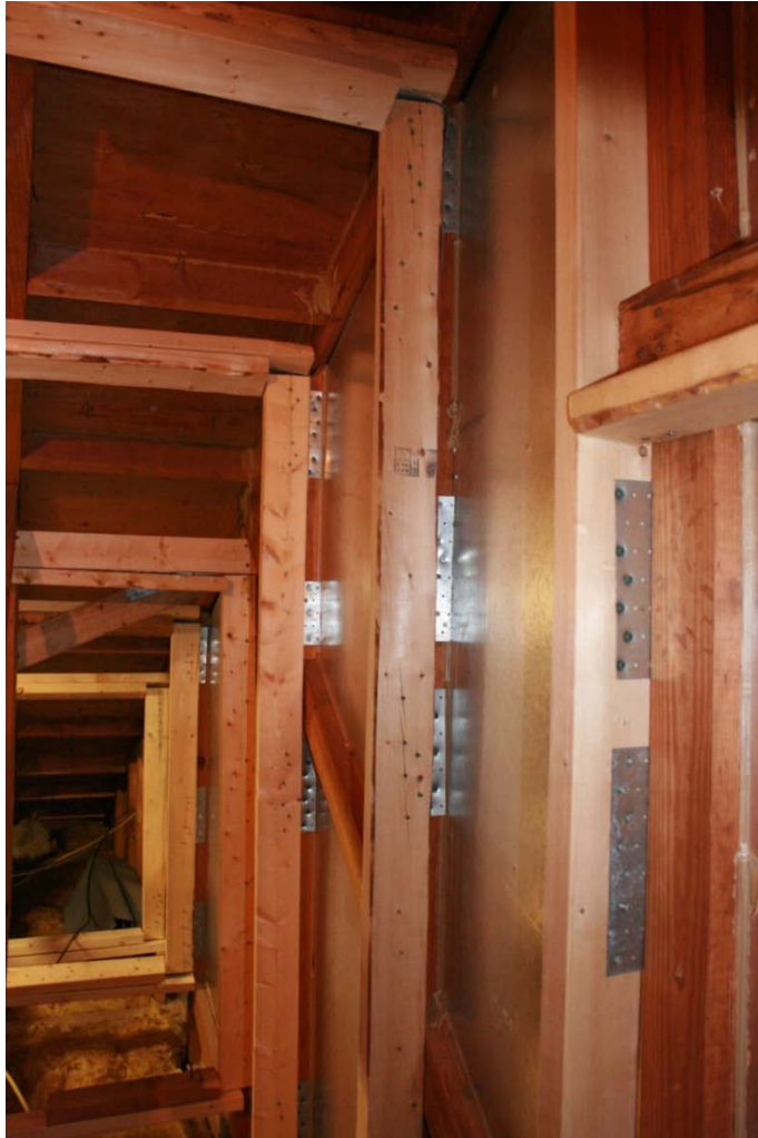
Figure 12.1. These show nail (nail, tie, mending) plates along the lengths of the retrofit and existing studs to bridge around webs on the truss.
