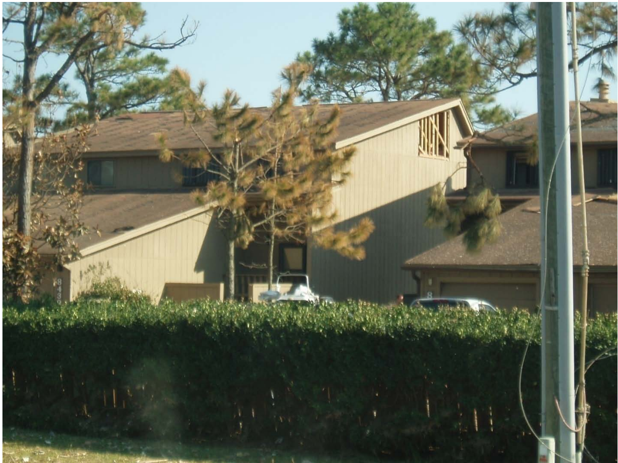
Figure 13.1. Missing siding pulled off by negative pressure or by wind that got into the house and pressurized it causing the siding to pop off. . If the wind shifted direction to blow rain into that opening, the damage to the rooms nearby could have been dramatic. Note plywood (or whatever) on the lower roof on the right.
