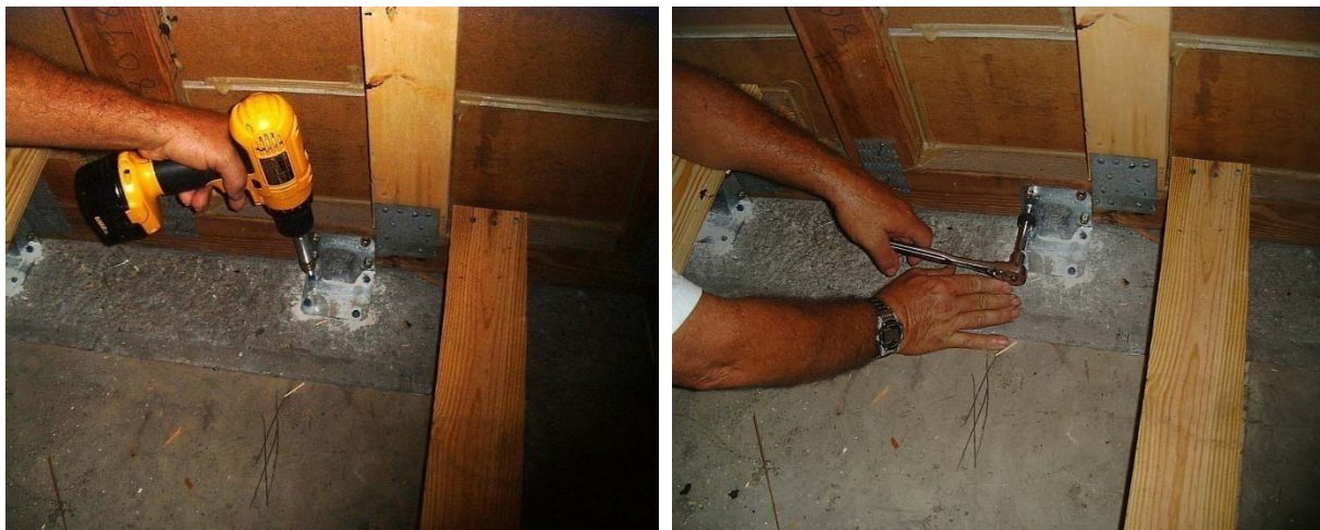
Figure 10.2. This shows an HGAM being installed directly to the top of the masonry wall. Here the elevation of the bottom chord was just fine as well as the grout in the concrete block being fine too.
