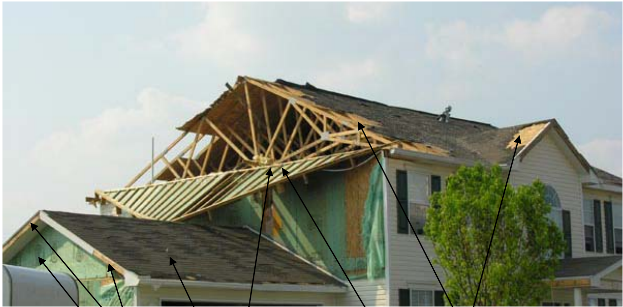
Siding blown off Fascia cover blown off Some shingles over garage blown off. The greatest damage and the reason for gable end retrofits. Gable end wall Some shingles blown off
