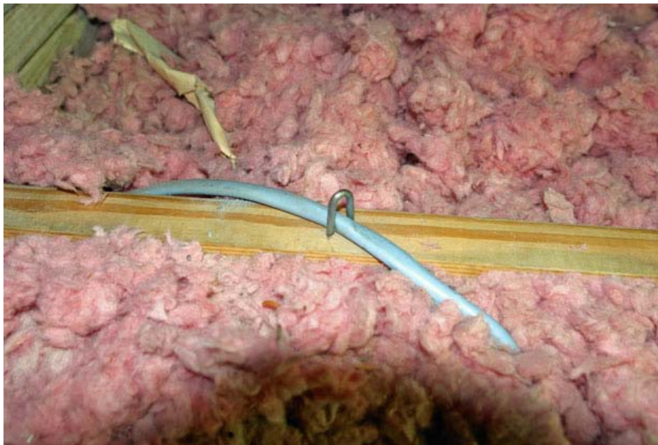
Figure 11.1. Electrical wiring running over ceiling joist. If the wire were to potentially be under a horizontal brace, the brace could be routed under it or the staple carefully removes and moved aside to avoid the conflict. Wires should NEVER sandwiched between horizontal braces and other framing members.
