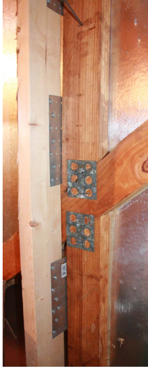
Figure 12.1. These show nail (nail, tie, mending) plates along the lengths of the retrofit and existing studs to bridge around webs on the truss.
