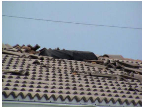
**This off-ridge vent broke loose - as a temporary repair, the owner put a tarp over it to minimize additional water leaks**
