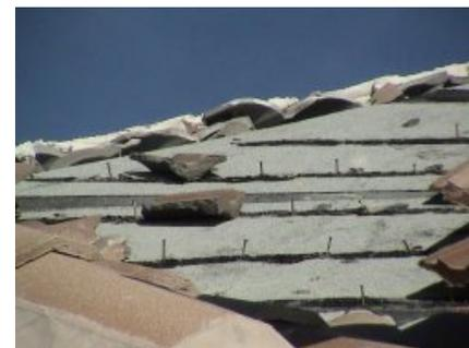
**Where the nails remained, they would plug the holes through the waterproof membrane under this tile roof - if any pulled out, they could leave small holes**
