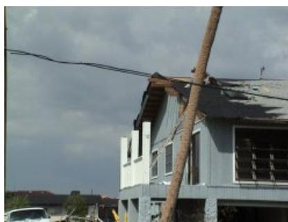
**Temporary repairs to reseal the edge of this roof that lost the porch overhang as well as roof cover on the main part of the roof**
