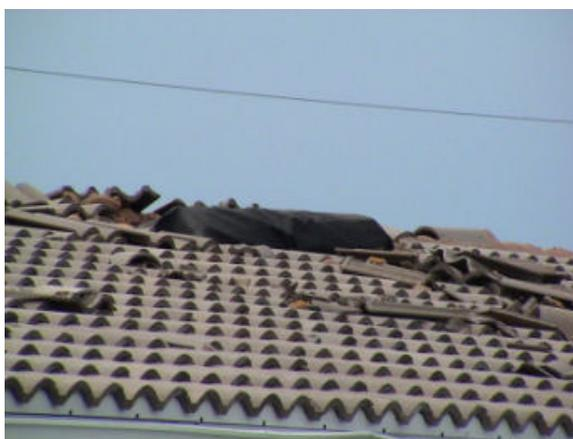
**This off-ridge vent broke loose - as a temporary repair, the owner put a tarp over it to minimize additional water leaks**
