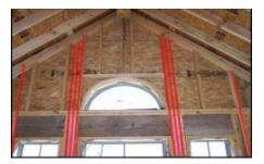
Gable end wall with cathedral ceiling - note The red lines indicate where continuous wall the horizontal joint running across the wall just below the semicircular window. The arrows point to where this wall is apt to fail in strong winds. Because there are no continuous vertical members crossing the indicated line, that line becomes a hinge point where the wall is likely to buckle.
