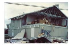
An example of the second most common type of gable end failure - the connection between the rectangular and triangular walls – It is rare that you actually find one that looks like this because usually the wall below fails and the whole end collapses. (click image for larger version)
