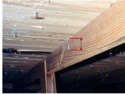
A shiner through wood plank roof sheathing
