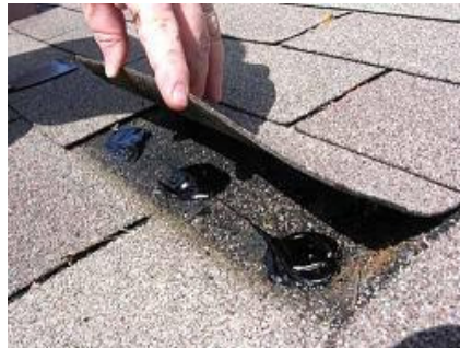
Applying dabs of asphalt adhesive under shingles tab (Hand Tabbing) (click image for larger version)
