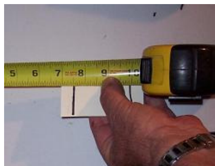
Determine the thickness of your roof sheathing
