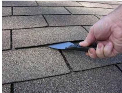
Breaking loose a partially adhered shingle to allow hand tabbing (click image for larger version)
