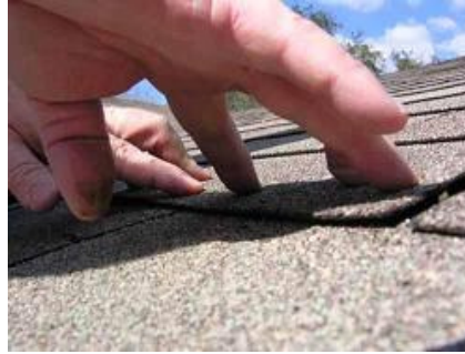
Pressing tab back against roof after applying dabs of asphalt adhesive
