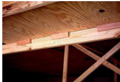
You can also get similar improvements in uplift using blocks of wood with adhesive on two sides
