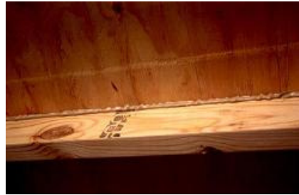
Bead of adhesive applied along the intersection between roof sheathing and rafters or truss top chord
