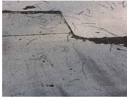
Patch on a section of membrane roof (click image for larger version)
