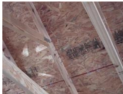
Oriented strand board roof deck
