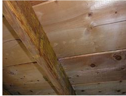
Planking roof deck
