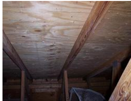
Plywood roof deck
