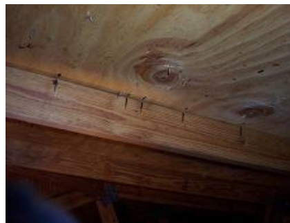
Marks showing locations of fasteners
