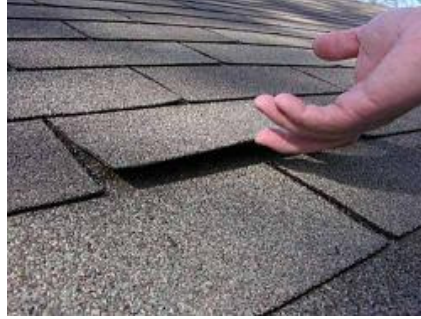
Loose shingle tab (click image for larger version)
