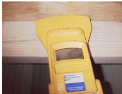
Using metal detecting stud finder to locate fasteners in rafters or truss top chords
