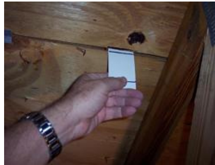
Using heavy paper to measure roof deck thickness
