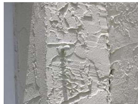
Stainless Steel Threaded Rod Epoxy Grouted Permanent Anchor with Cap
