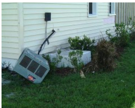
A couple of angle brackets could have kept this compressor in place
