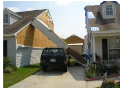
This chimney box was only attached with a couple of toe-nails near the roof
