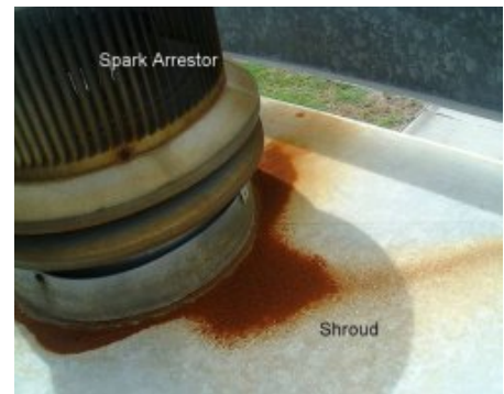
Spark arrestor showing minor rust
