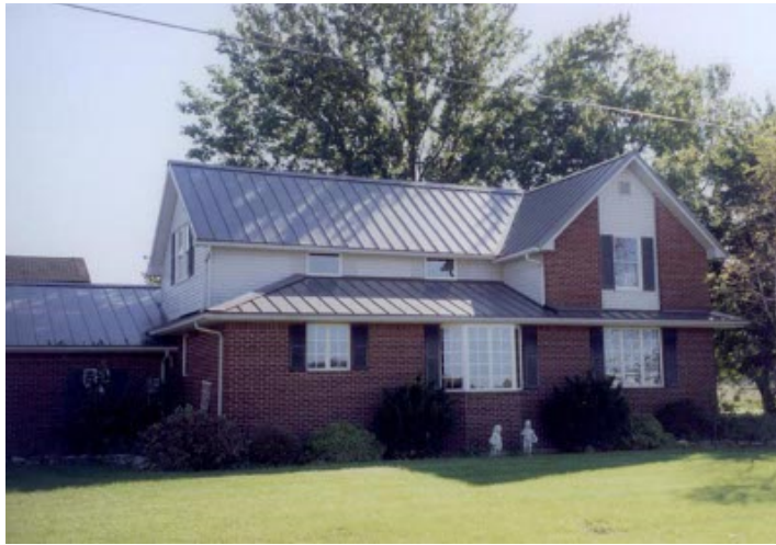
Standing seam metal roof
