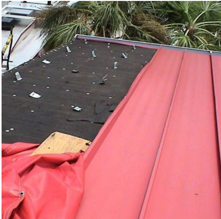
Standing-Seam metal roof with missing panels - note shiny clips that are curled into the seam between the metal panels
