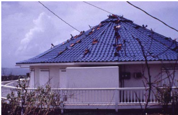
Typical hurricane damage to metal tile roof
