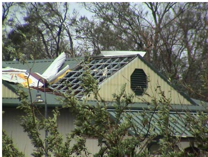
Metal roof without deck - when the metal lifts off, the interior of the building is exposed
