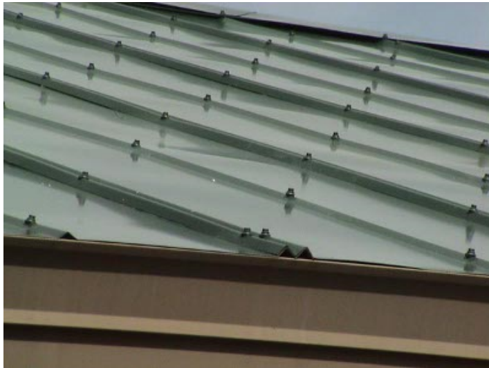
5-V Crimp metal roof with external fasteners - makes it easy to see how well the metal is anchored to the roof deck
