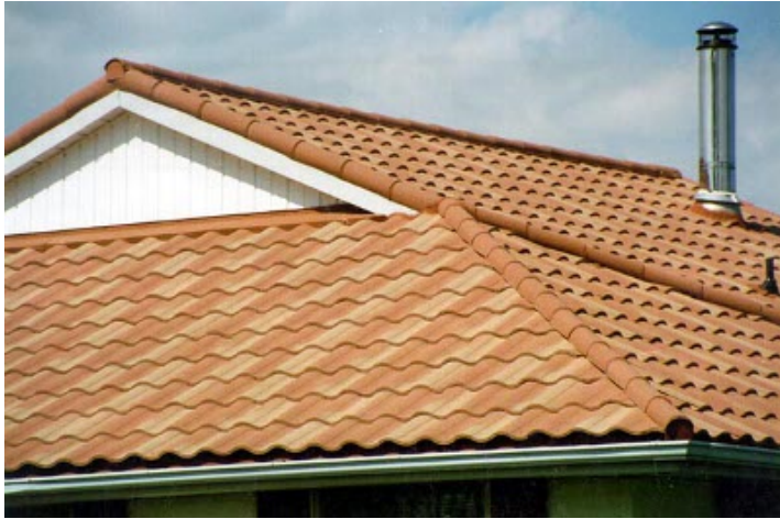
Metal roof made to look like tile
