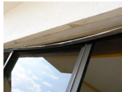
A track anchorage failure for a set of sliding glass doors. Note the single fastener hole above the door panel.
