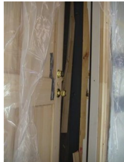
This un-reinforced door frame gave way at the strike plate when the door was subjected to wind pressures. The vinyl sheeting was used to help apply the pressure.
