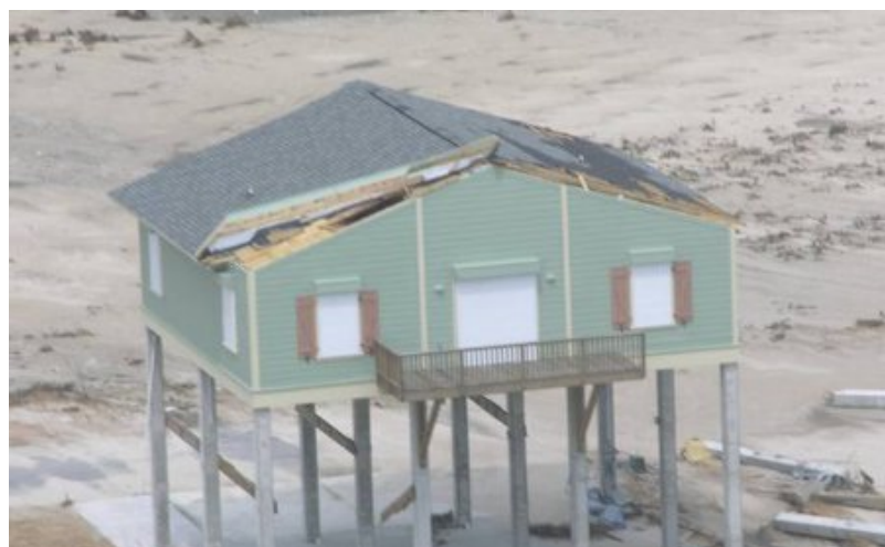
Gable End Roof Sheathing Damage From Outlooker Connection Failure: The Gable Overhang on the Left Side of the Roof Flipped Onto the Roof
