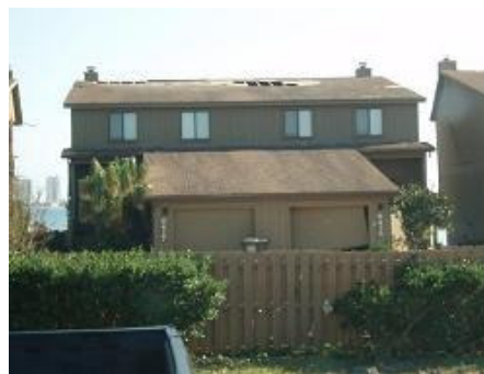
Missing panels from the middle of roof indicates poor nailing of sheathing.
