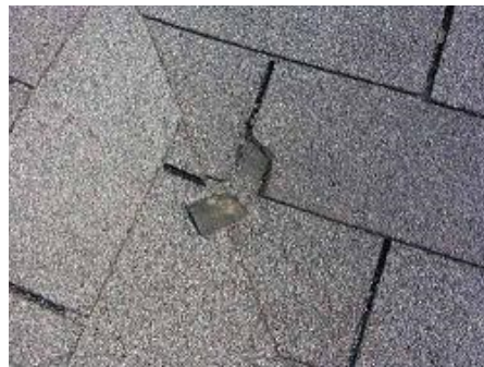
Broken Shingle Tab
