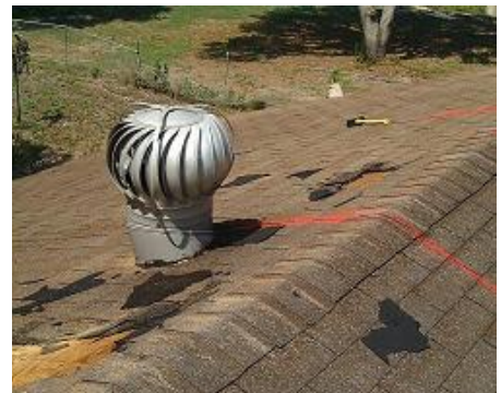
Roof Ventilation Turbine
