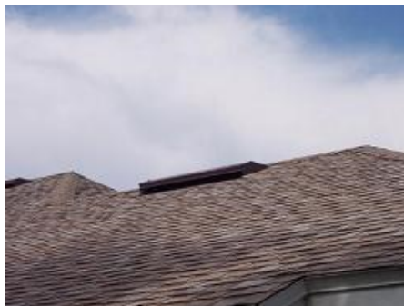
Off-Ridge Vent on Shingle Roof
