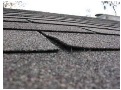
Partially Lifted Shingle Tab
