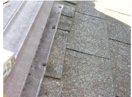
Ridge Vent Connection to Roof with Nails Working Their Way Out a Very common occurrence
