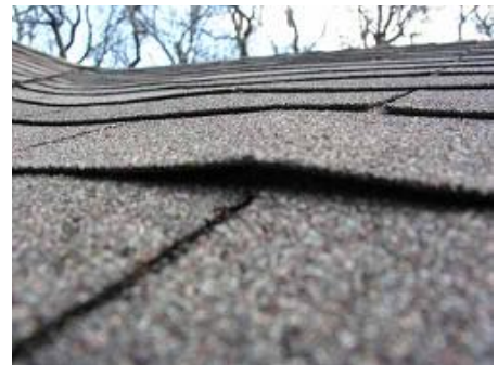
Buckled Shingle Tab
