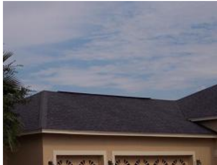
Ridge Vent on Shingle Roof
