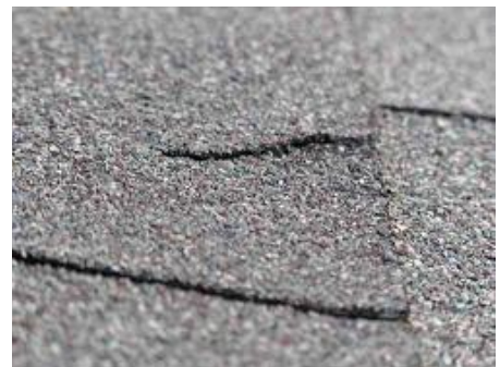
Cracked Shingle Tab
