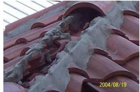
**Close-up of ridge tile showing anchorage at edges using mortar - hollow cavity**
