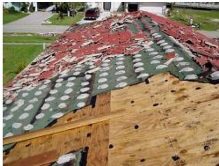
**Mortar set tiles rely on adhesion of tile to mortar and mortar to underlayment**
