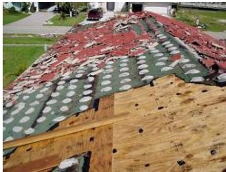
**Mortar set tiles rely on adhesion of tile to mortar and mortar to underlayment**
