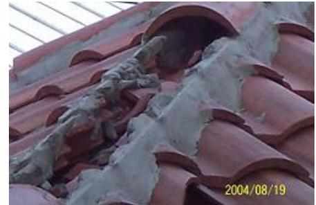
**Close-up of ridge tile showing anchorage at edges using mortar - hollow cavity**
