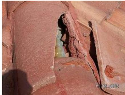
**Ridge tile (note adhesive never made contact with metal hip/ridge frame and minimal contact of adhesive at the tile overlap at the bottom of the ridge tile)**
