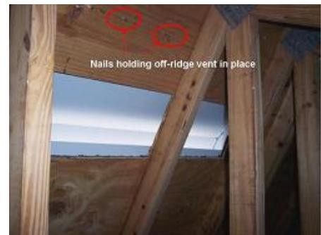
**Off-ridge vents on tile roof house. The covered vent broke loose and allowed a tremendous amount of water to enter the house**
