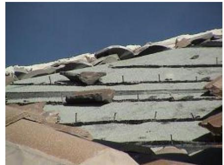
**Mechanically attached tile - most of the tile failure was probably caused by impact of tile from a neighbor's house, but in some cases there were indications that the tile worked its way off the head of the fastener**
