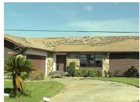
code requirements (at least in Florida) and industry recommendations call for attaching the hip/ridge tiles to a wood or metal hip/ridge board or cap using screws and adhesives, nails and adhesives, adhesives only or nails and possibly clips.
