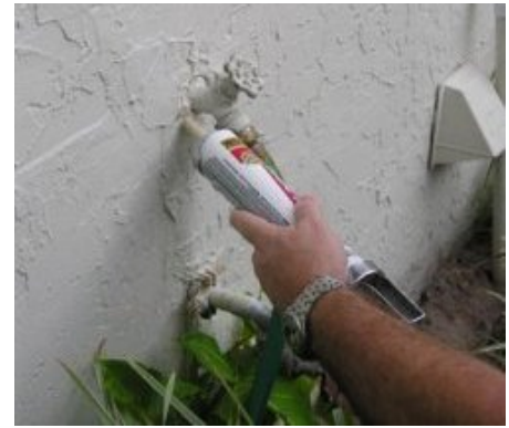
Sealing gaps and cracks around an outdoor hose bib
