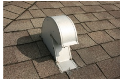
Gooseneck vent for bathroom or dryer exhausts.
