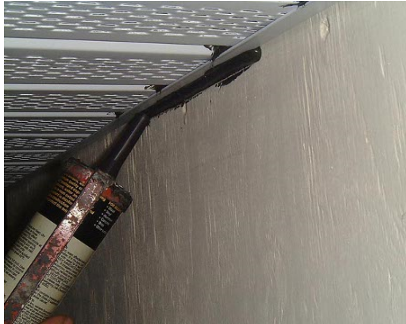
Caulking bottom edge of soffit wall J track to wall to improve anchorage of track – black caulk shown for contrast.
