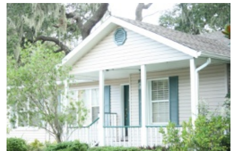
This shows an appliqué type vent that may be functional or decorative
