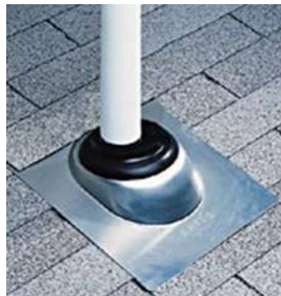
This vent pipe flashing fits snugly around the pipe preventing water from getting into the attic.
