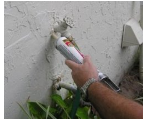
Sealing gaps and cracks around an outdoor hose bib
