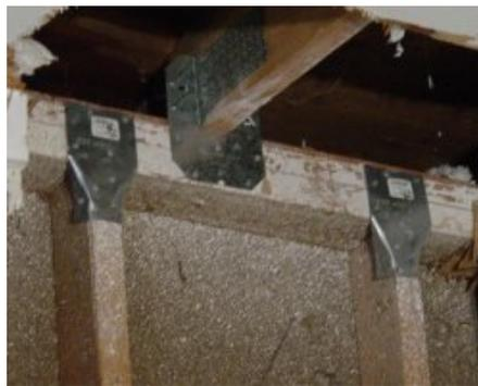
**You can use a combination of straps to transfer uplift from the trusses or rafters through the double top plate and into the wall studs. The more structure you can engage in resisting the uplift, the better. This photograph shows two sets of connectors. The top one connects a truss or rafter to the top of the double top plate**
